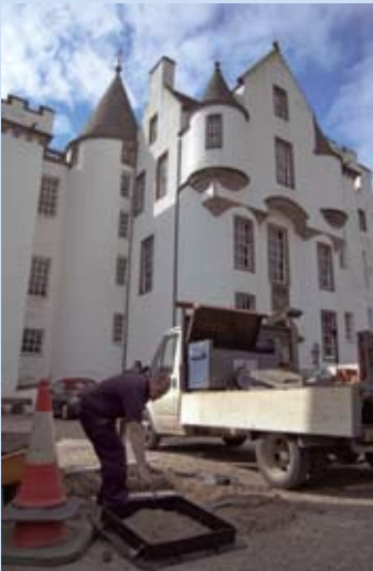
Andrew Jackson repairing a forecourt service duct cover
